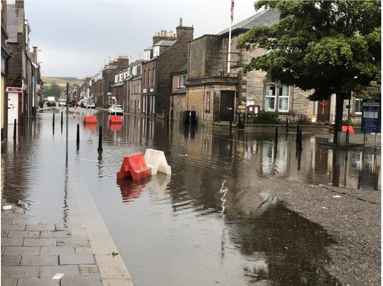
Figure 5: Flooding of Barclay Street, Stonehaven on the 12 August. Source: SEPA
